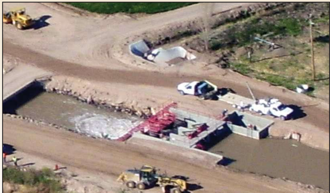
EBID completes construction of experimental bypass turbine box at Station 8.
