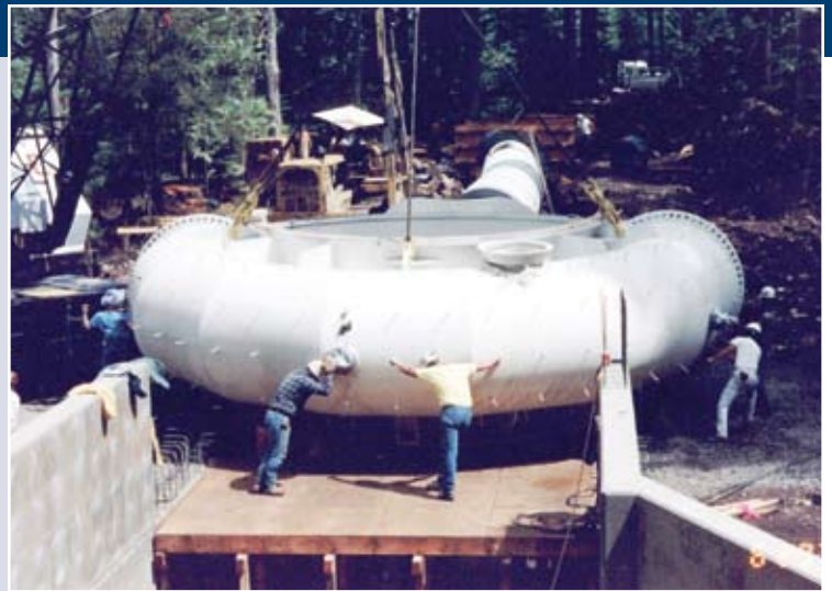
Scroll Case being set and connected to penstock for Francis turbine.
