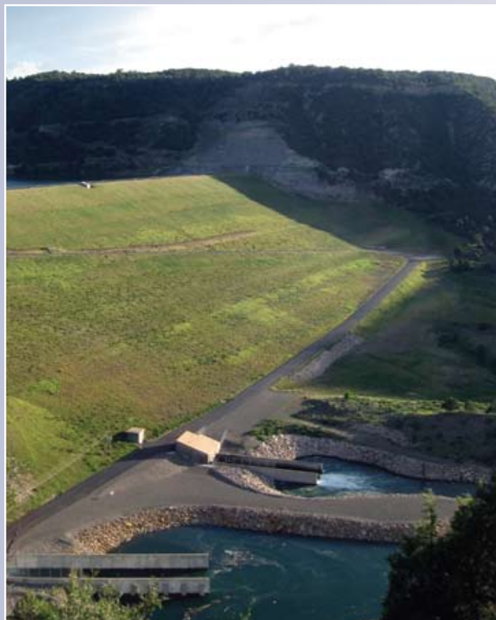
Ridgeway Dam, Colorado: Proposed site for 7 megawatt hydropower plant.
