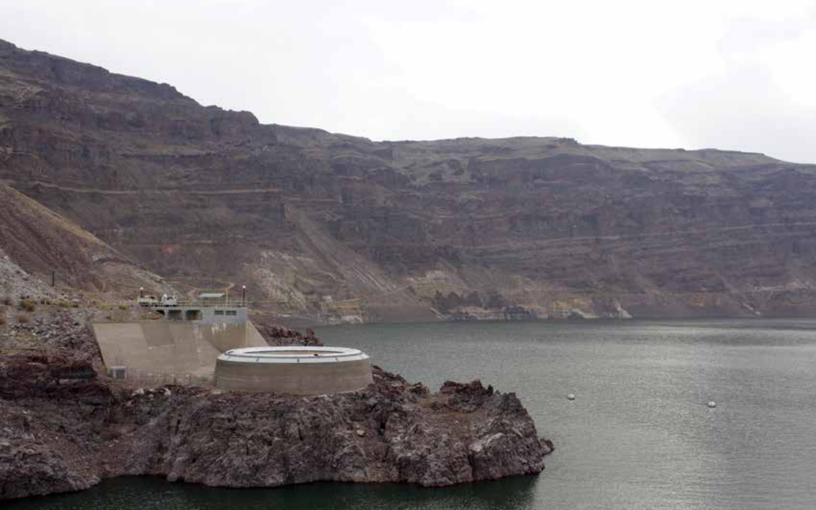
Ring Gate, Owyhee Dam Spillway.
