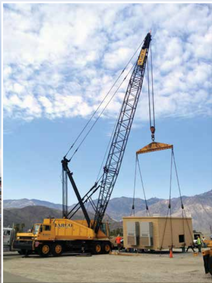
Craning in a prefabricated concrete block building.
