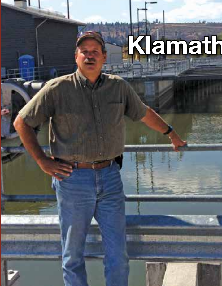
Mark at KID's headworks and fish screen facility at "A" Canal.
