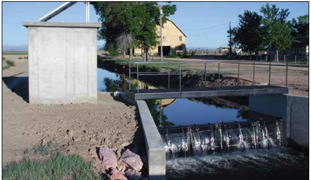
Check structures on the Larimer Weld Irrigation Canal in Colorado. The Obermeyer Gate System facilitates controlled water diversion at rivers without fluctuations in diverted flow caused by river flow changes.
