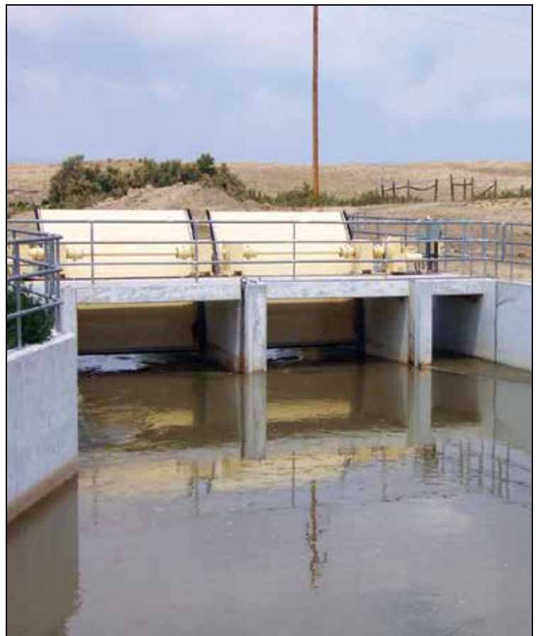
One of the check structures funded in part by fish recovery money.
