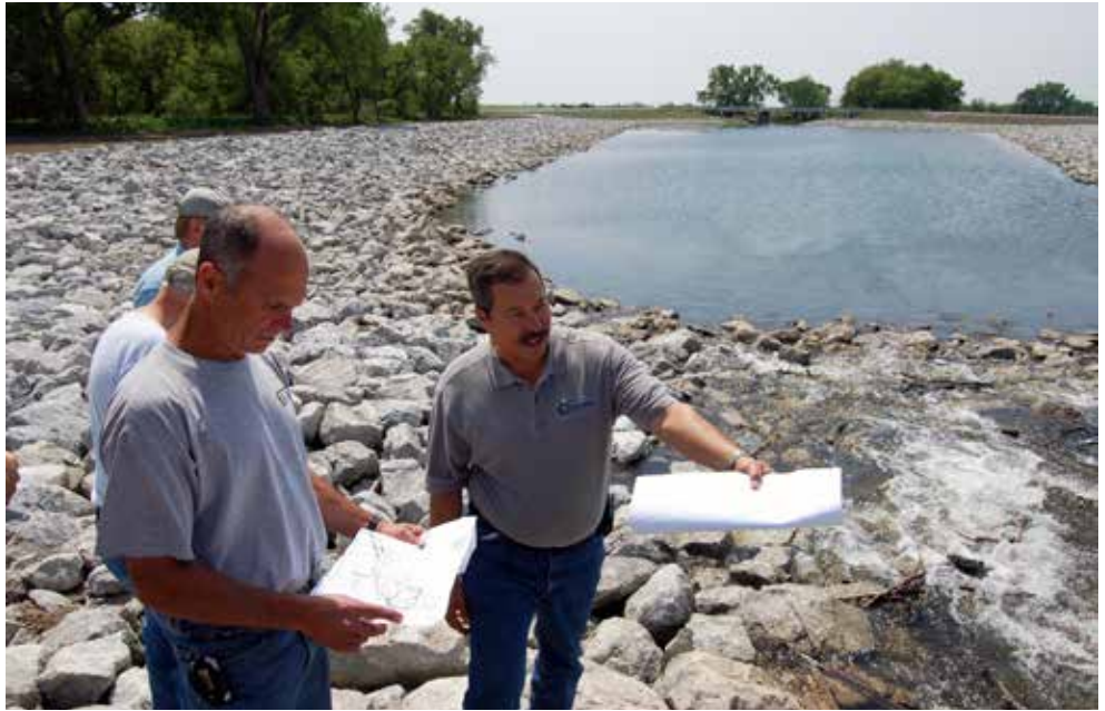
John Miyoshi explains the wetland retention structure to Lower Platte North NRD staff above Lake Wanahoo in 2009.
