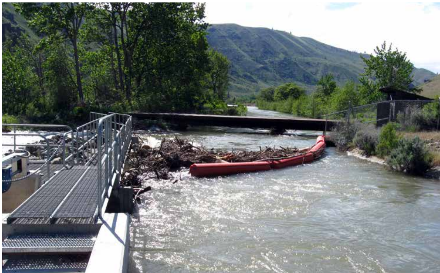
Naches River diversion. The TUFFBOOM protected facilities during a flood event, helping to maintain canal diversion flows.
