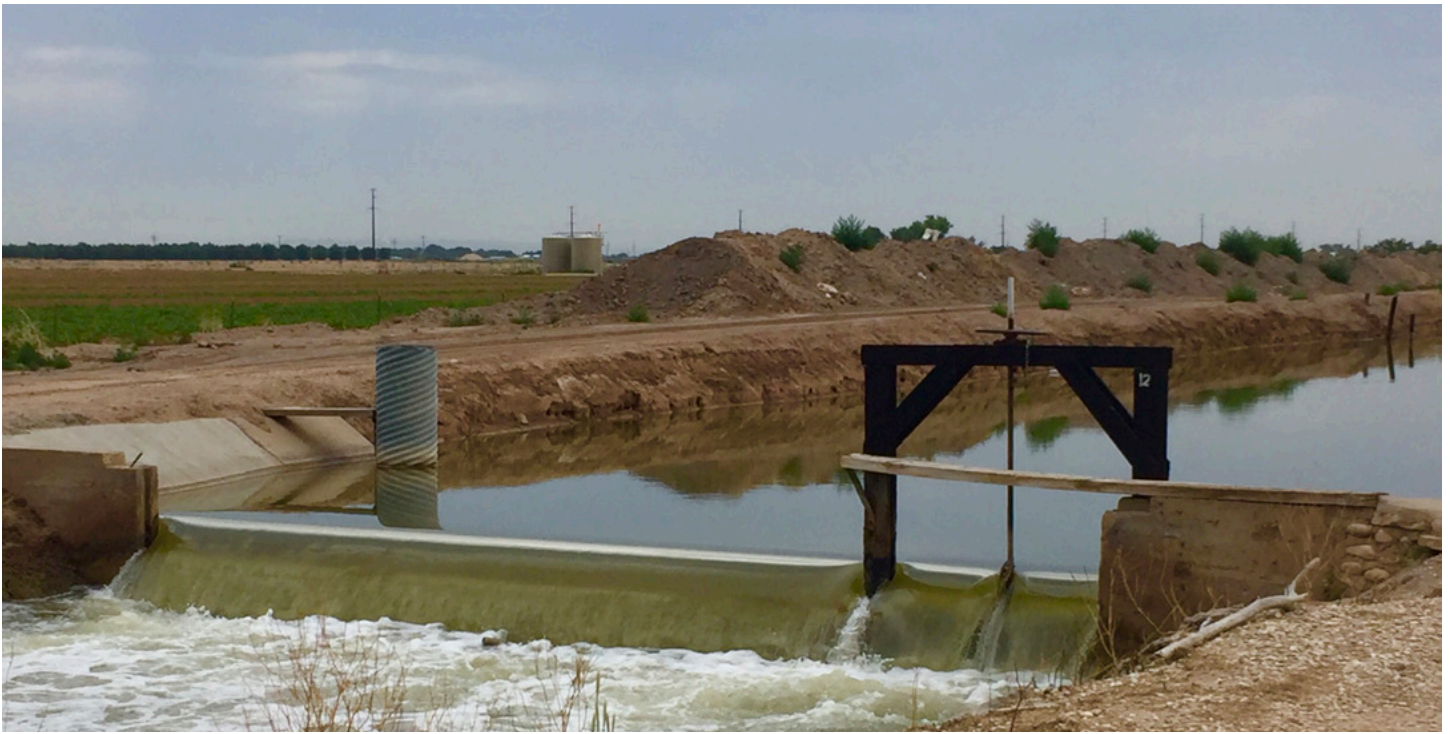
The main canal at CID's lateral 12.
