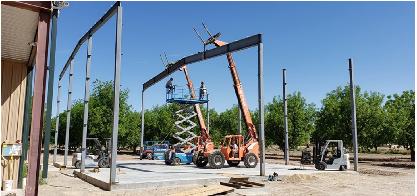
Dixie Ranch's freezer building under construction.
