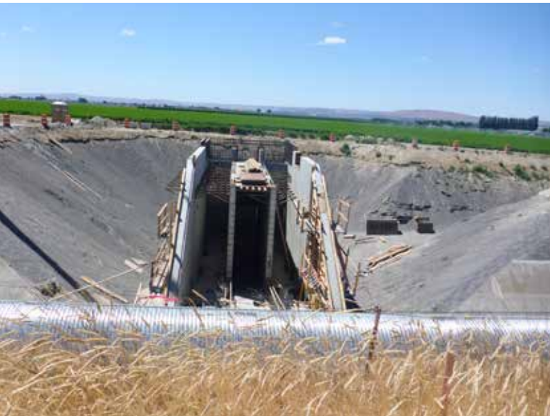
South Columbia Basin Irrigation District's Esquatzel pumping plant under construction.
