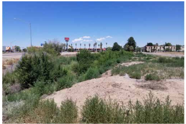
The Park Drain before cleaning.
