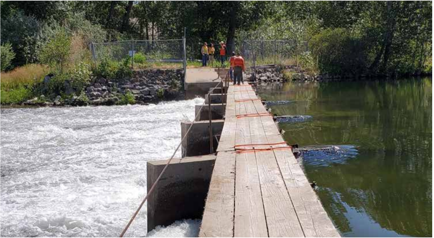
The Ridenbaugh Canal check structure in use in July 2019.
