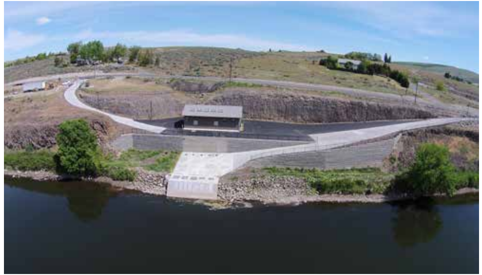
The Kiona pump station and intake at KID's Red Mountain Local Improvement District.
