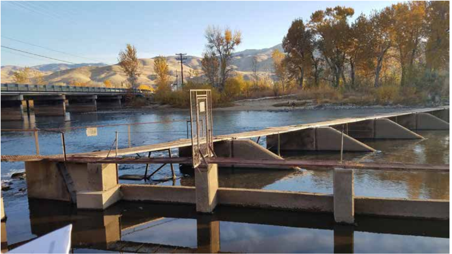
The Ridenbaugh Canal diversion check structure on the Boise River.
