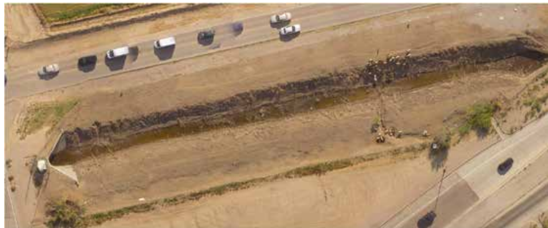
The Park Drain, eaten clean of overgrowth.
