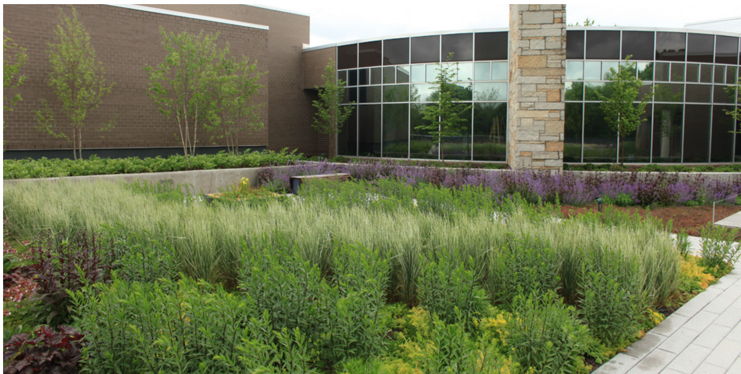
The green roof at the Frederik Meijer Gardens and Sculpture Park was a joint effort among the owners, the architects, and LiveRoof.
