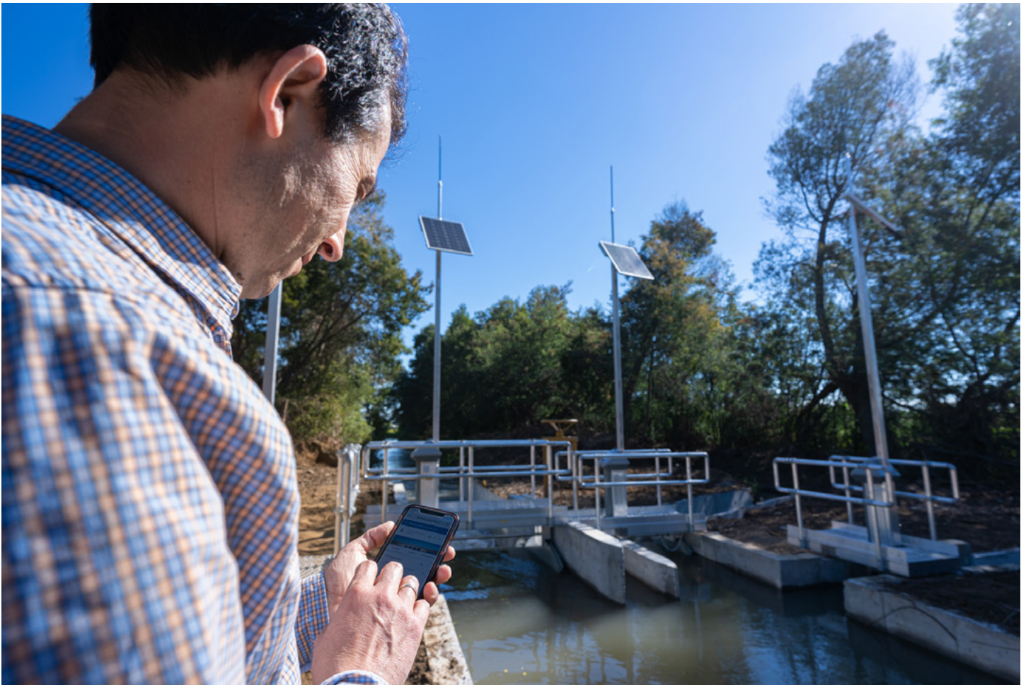
Rodrigo Romero Jara, the manager of the North Biobío Canal Association in Chile, operates a Rubicon gate.
