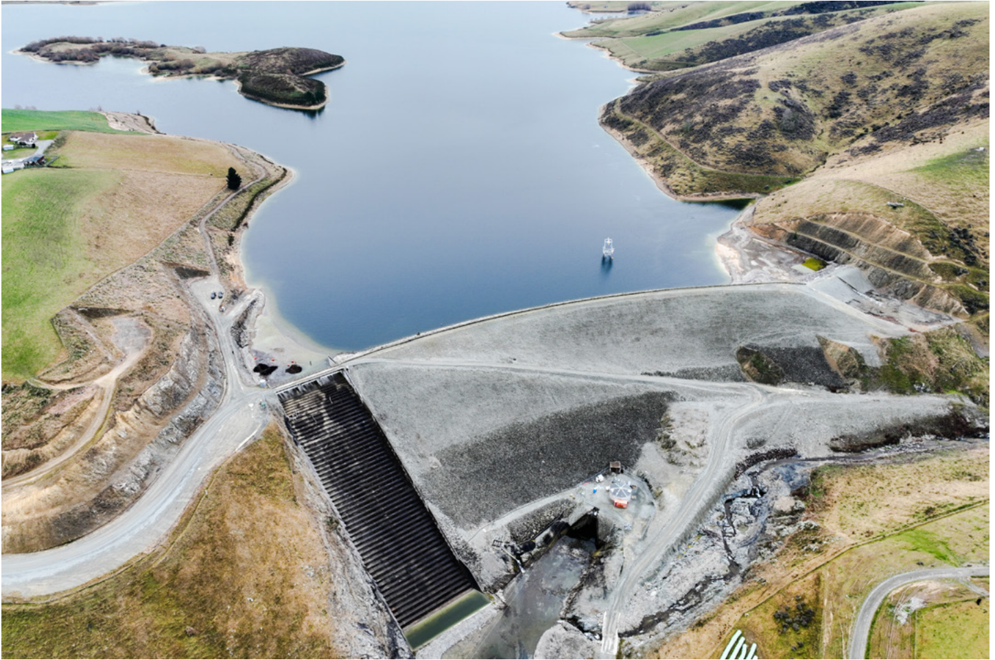
An aerial view of Opuha Dam and Power Station, winter 2022.
