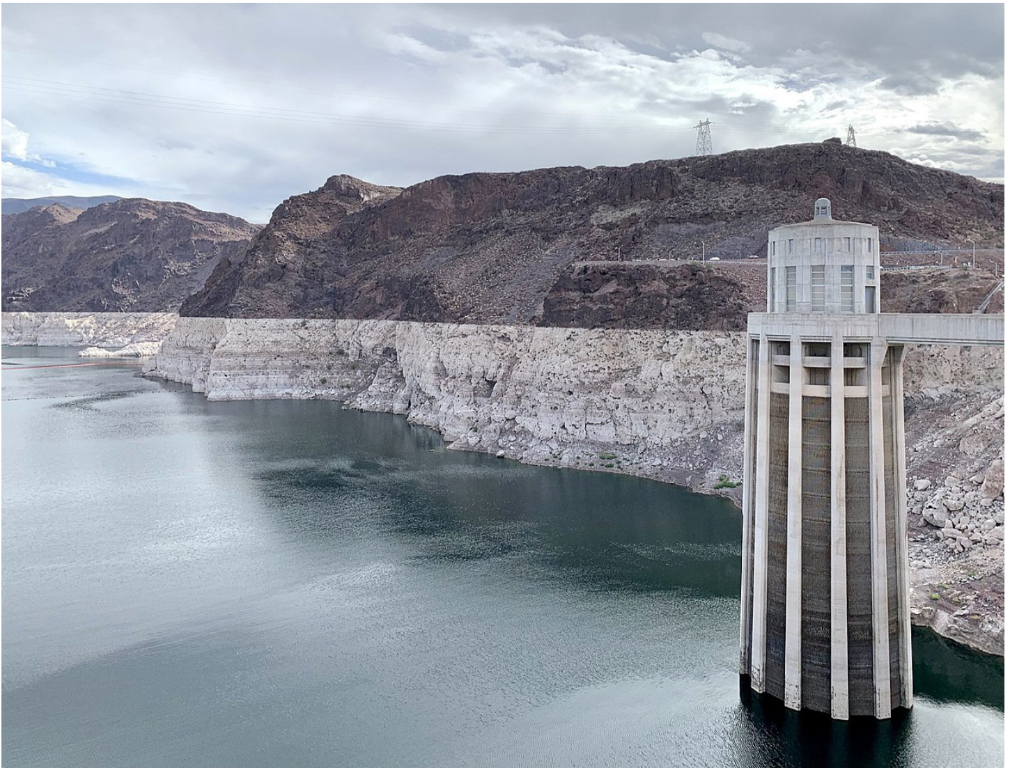
A water intake at Hoover Dam in October 2021, when water levels were approximately 20 feet higher than they were a year later.
