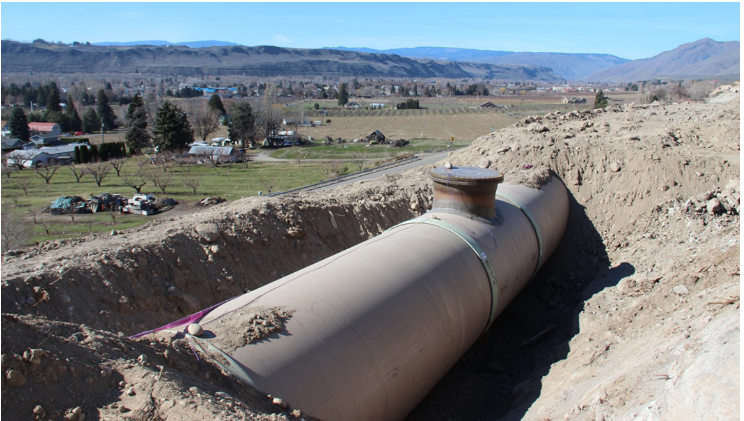
Hobas pipe in a flume at Washington State's Naches-Selah Irrigation District.
