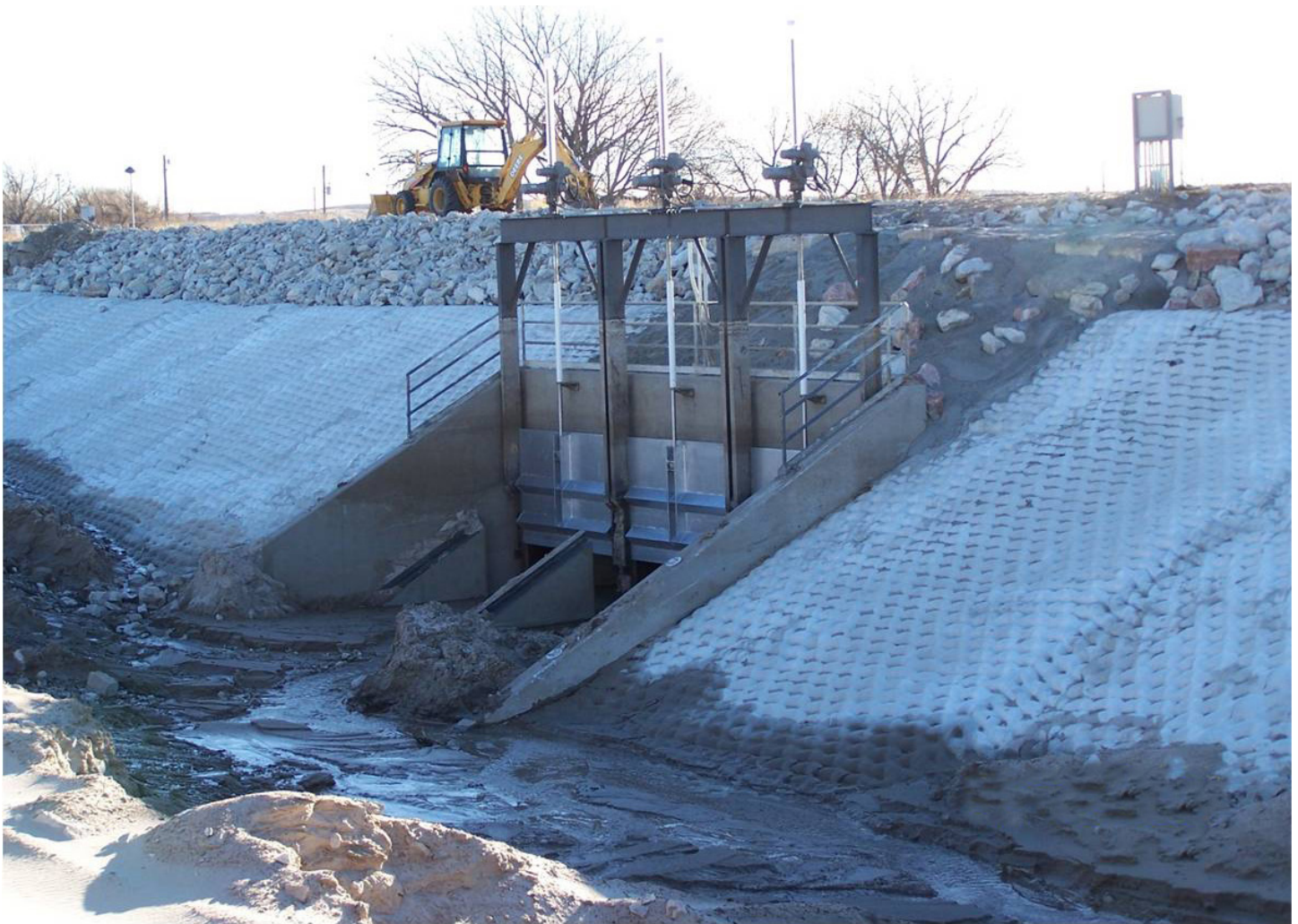
Construction on Milburn Dam in 2007.
