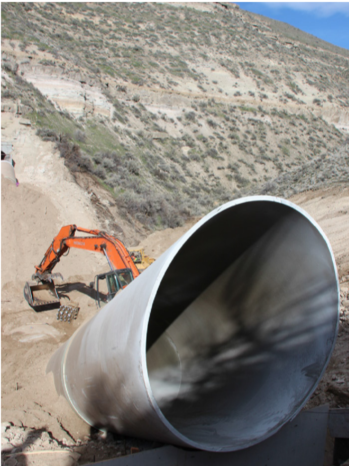
HOBAS supplied a custom-built 96-inch pipe tee along with two custom elbows to create a V-shaped siphon for the Naches-Selah Irrigation District. It also supplied 3,600 feet of 96-inch pipe.
