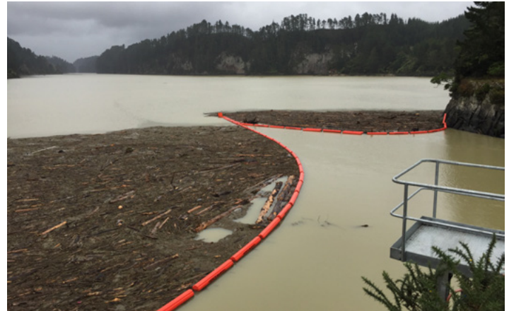
A Worthington-designed debris boom deflected debris away from the spillgates and water intakes at Matahina Dam in New Zealand after an extreme rainfall event.
