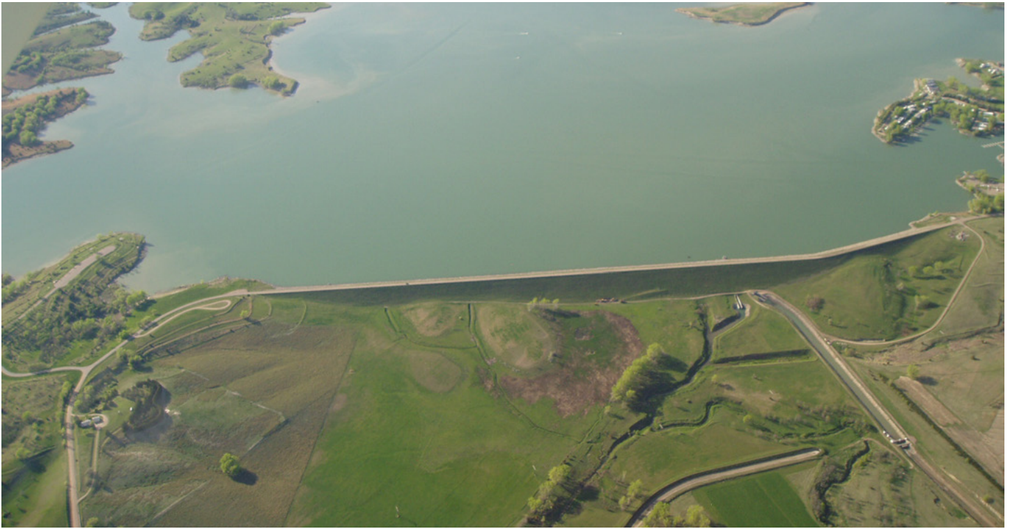
Sherman Dam and Reservoir.
