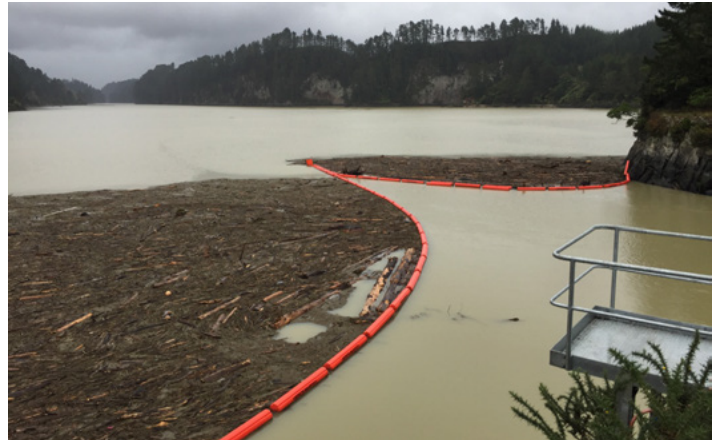
A Worthington-designed debris boom deflected debris away from the spillgates and water intakes at Matahina Dam in New Zealand after an extreme rainfall event.
