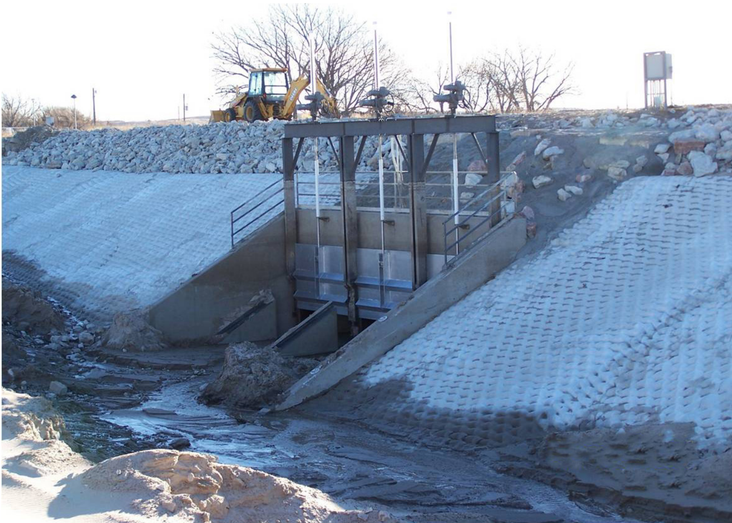
Construction on Milburn Dam in 2007.
