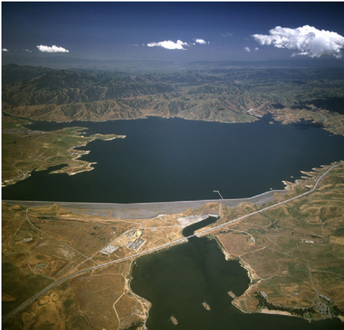
The B.F. Sisk Dam raise, which will benefit from Bipartisan Infrastructure Law funding, will add 130,000 acre-feet of storage.
