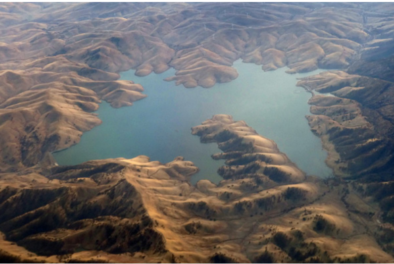
The expansion of Los Vaqueros Reservoir, which will benefit from BIL funding, will add 115,000 acre-feet of storage.
