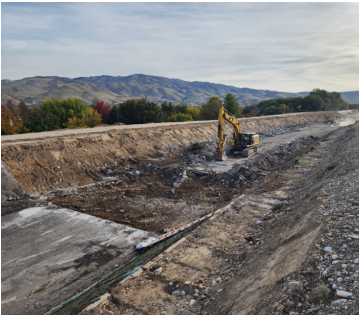
The board of control has to remove every bit of the existing liner before it relines.
