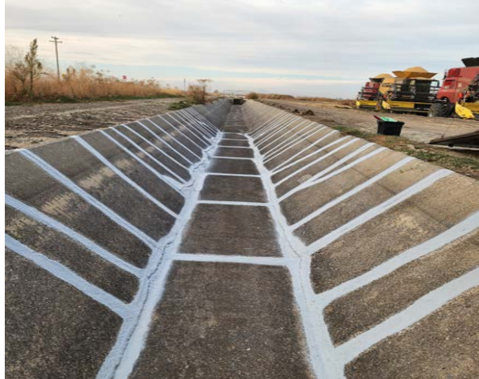
A concrete-lined canal sealed with AquaLastic.
