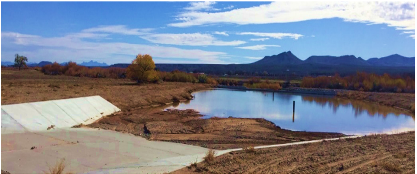
The Thurman Arroyo II sediment interception basin, located along the Rio Grande near Hatch, New Mexico.
