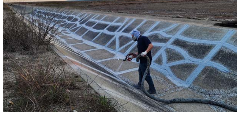
AquaLastic is applied to an RD108 canal.
